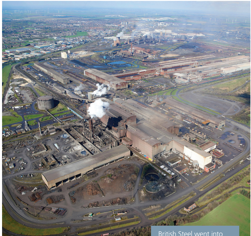
British Steel went into liquidation in May 2019, putting 25,000 jobs at risk
